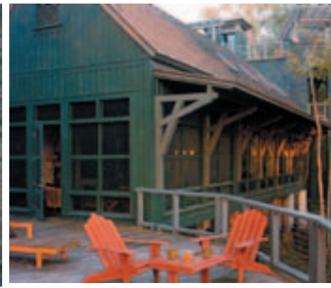
Decks, screened porches, and balconies all reinforce a connection to the outdoors. The dark color palette provides a complementary addition to the natural setting.
