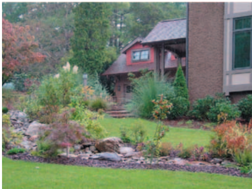
Dry Creek Beds or Water Quality Swales can be used to slow the flow of stormwater and allow for infiltration of rainwater into the ground. This system also treats and filters stormwater, improving water quality and minimizing the potential of sedimentation from reaching nearby streams.
