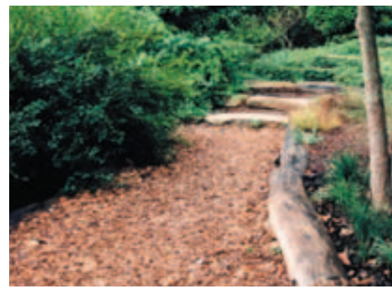
The mulched path illustrates the appropriate use of materials for pathways and trails. Decomposed granite is also appropriate for trails. Stone and chip seal are appropriate materials for pathways.
